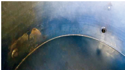
Bottom of bulk storage tanks after cleaning.
