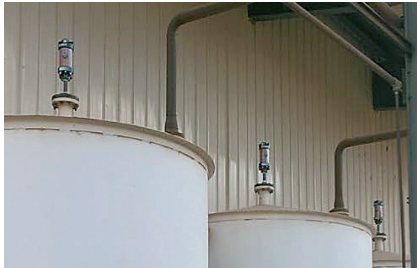
Bulk storage tanks refitted with desiccant breathers.
